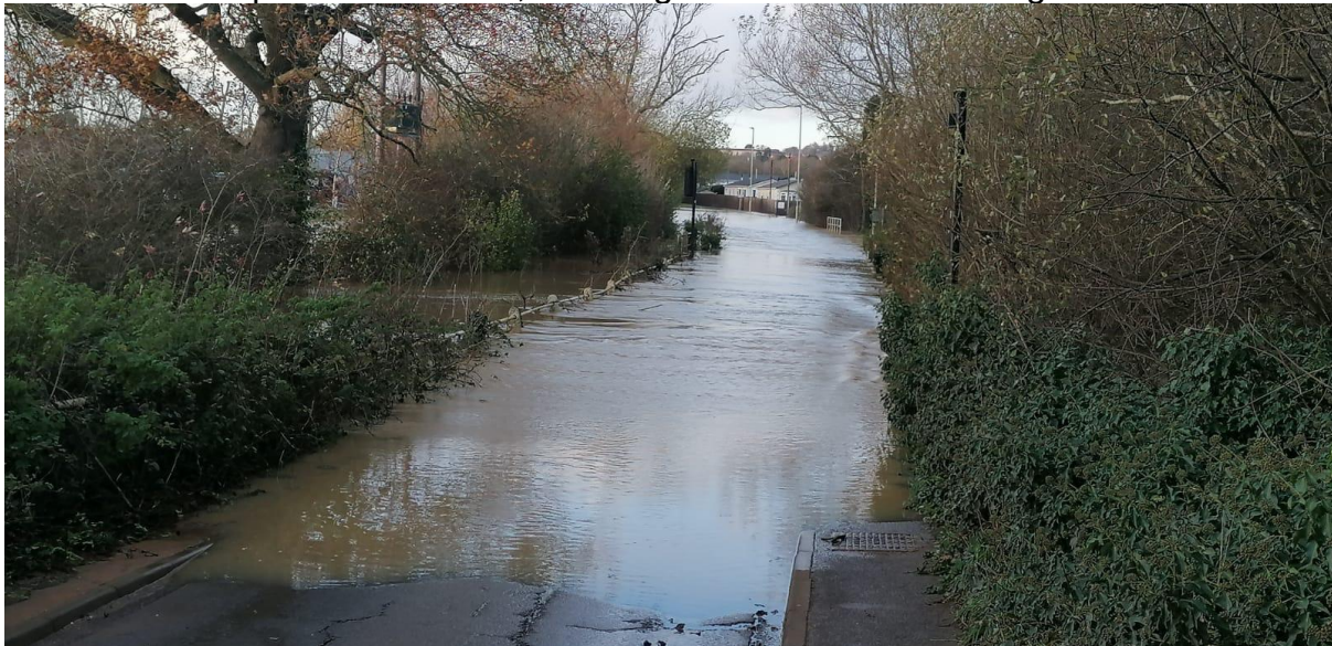
The approach road to the bridge closed due to flooding
