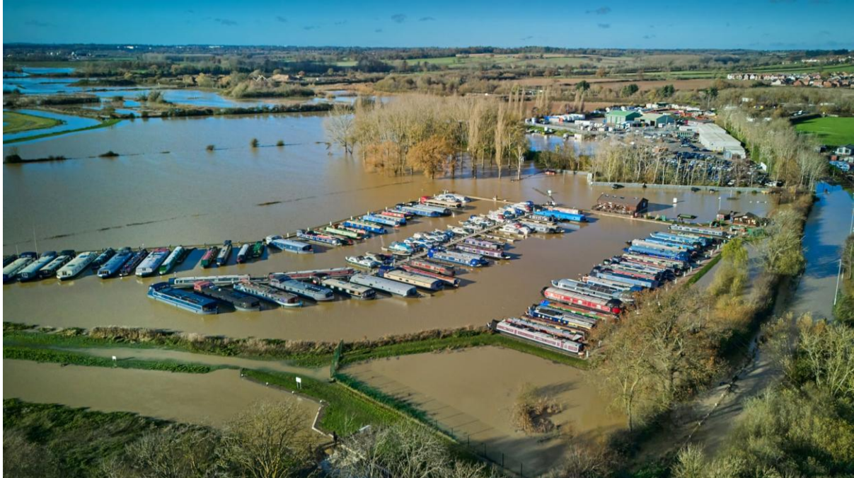
The Marina car park under water, the bridge closed due to flooding November 2024
